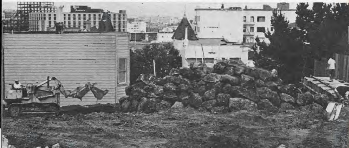
Park construction—the pile of boulders is a climbing structure connected to the concrete slide.
